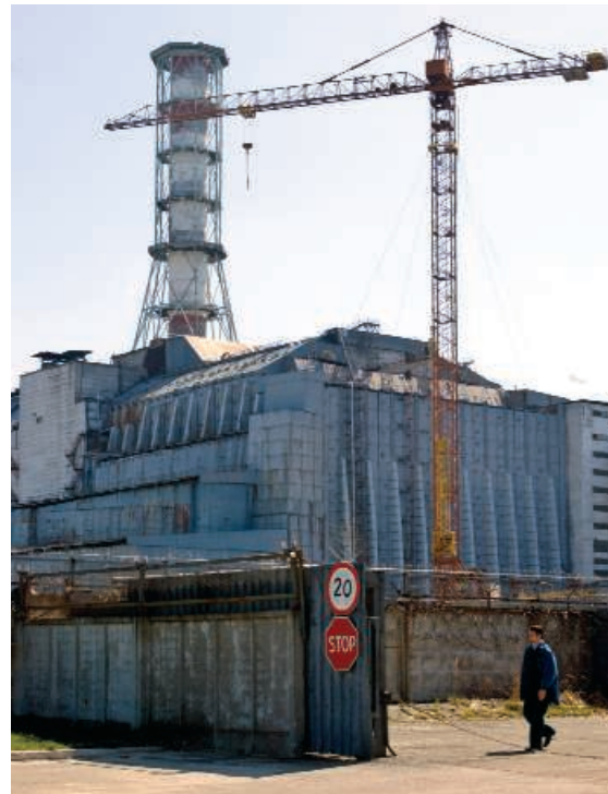
Sleeping giant. A guard walks past the remains of Chernobyl’s reactor #4, which is encased in a now-crumbling sarcophagus.
